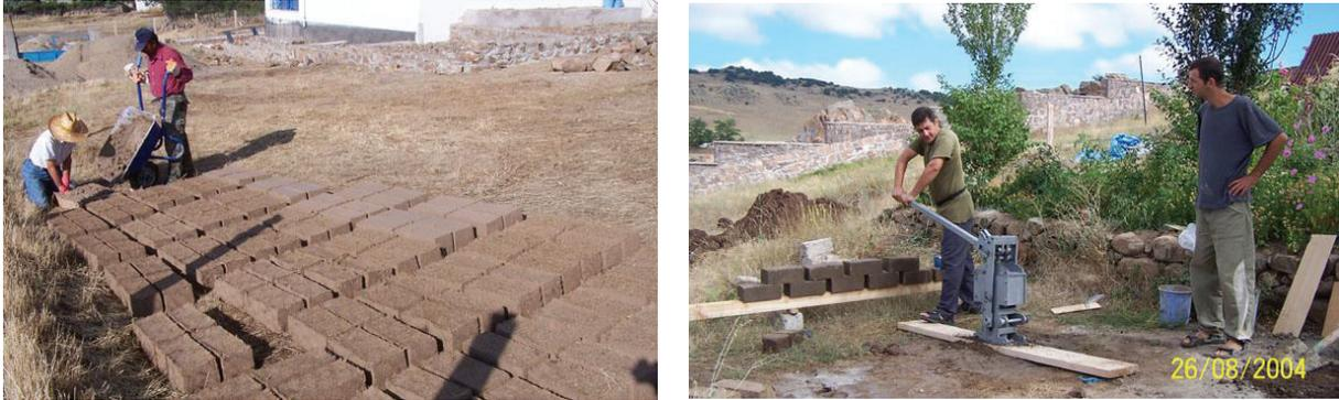
Figure 9. Traditional sun dried mudbricks (left) and pressed bricks (right) were produced at Kerkenes and used for small projects designed by students.
