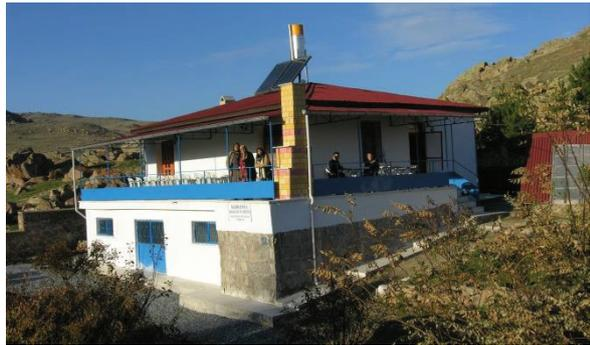
*Figure 6. The Erdoğan Akdağ Center was built with a concrete frame and AAC blocks infill.*
