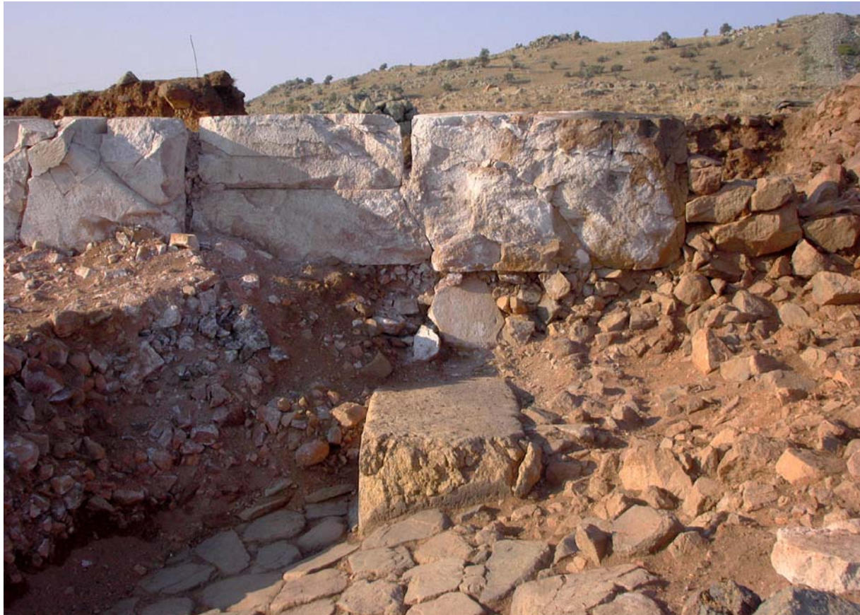
Figure 16. The north wall of the South Tower is structurally unstable due to the burning of horizontal timbers between the courses of large blocks. A large conglomerate plinth set into the granite pavement and trimmed in situ, may have been the base for a lion or sphinx. (04dpjv2512)
