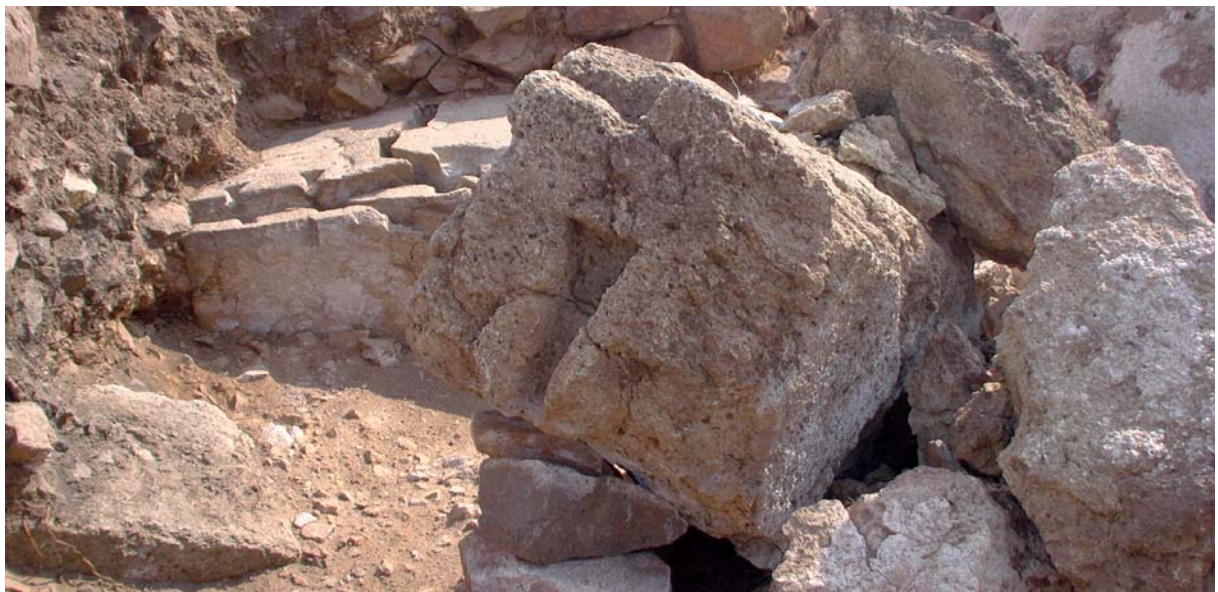
Figure 19. A fallen block of conglomerate has two clamp cuttings, that on the top left being incomplete. The granite block seen in Fig. 10 is in situ in the tower wall behind. (04dpjv2215)
