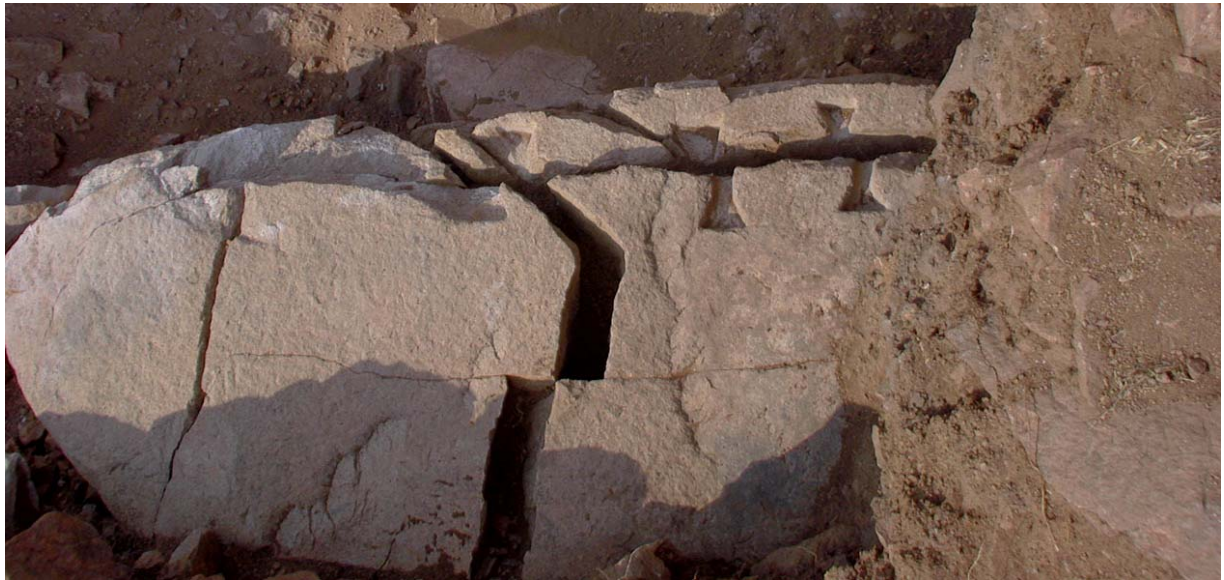
Figure 18. A row of small clamp cuttings for mending the front of a split granite block in the north wall of the South Tower. This is probably a corner stone, the end being just beyond the baulk at right. (04dpjv2219)
