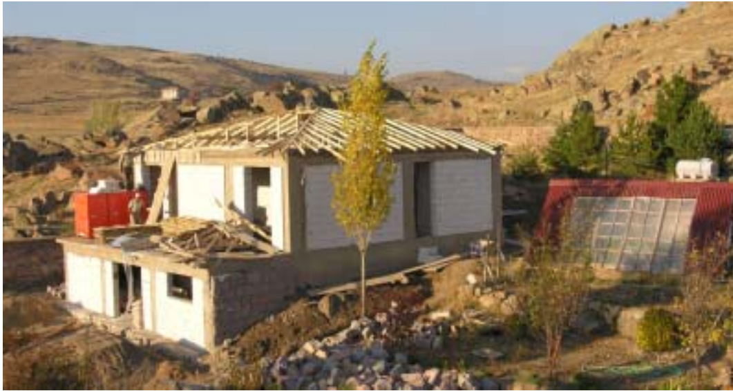
Figure 5. Construction of the Erdoğan Akdağ Center for Research and Education. AAC blocks, cement, sand and roofing sheets were donated by AKG Gazbeton, YL Yozgat Çimento, the Sorgun Belediye and Onduline respectively. (05kenc0628)
