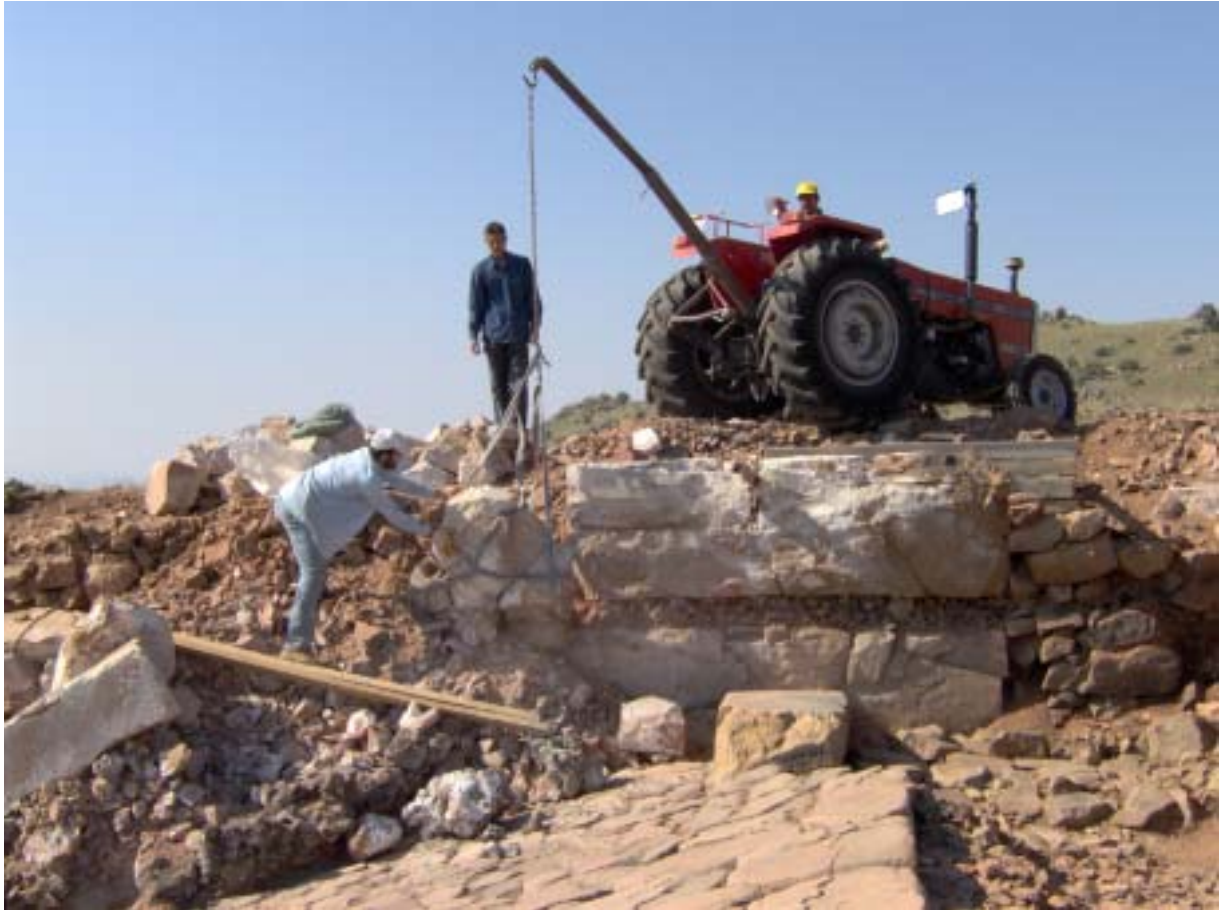
Figure 24. The horizontal gap left between courses after the horizontal beam completely burnt down caused the wall of the South Tower to become structurally unstable. Facing blocks and burnt debris are naturally coated with white carbonates. Many of the large stones, shattered by the intensity of the fire, had to be removed for safety. (05dphp1104)
