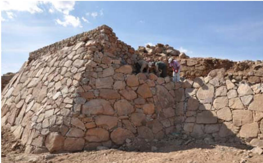
Figure 153. The glacis was rebuilt to its full height across the junction between the East Tower and the City Wall. (10dpnd1422)
