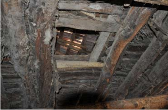
Figure 65. The original flat roof was constructed of beams supporting rafters covered with split branches and a thick layer of mud. A trap door cut through the original roof provides a glimpse of the recently added clay tile pitched roof. (10dpnd1905)
