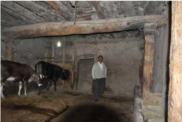
Figure 66. Kara Mehmet in his stable, now used as a cowshed, at Şahmuratlı village. A central drain runs the length of the concrete floor while food troughs run down either side. The doorway at the far end leads into a dry store for fodder. Note the size of the juniper roof beams which are no longer available in the immediate region today. (10dpnd1904)
