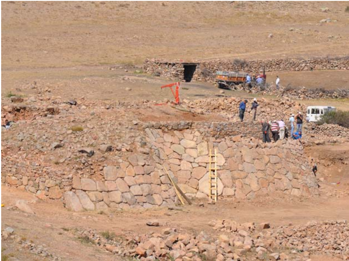
Figure 130. Stones, previously cleared from around the Gate structure and dumped nearby, were used to restore the glacis. (10dpnd1121)
