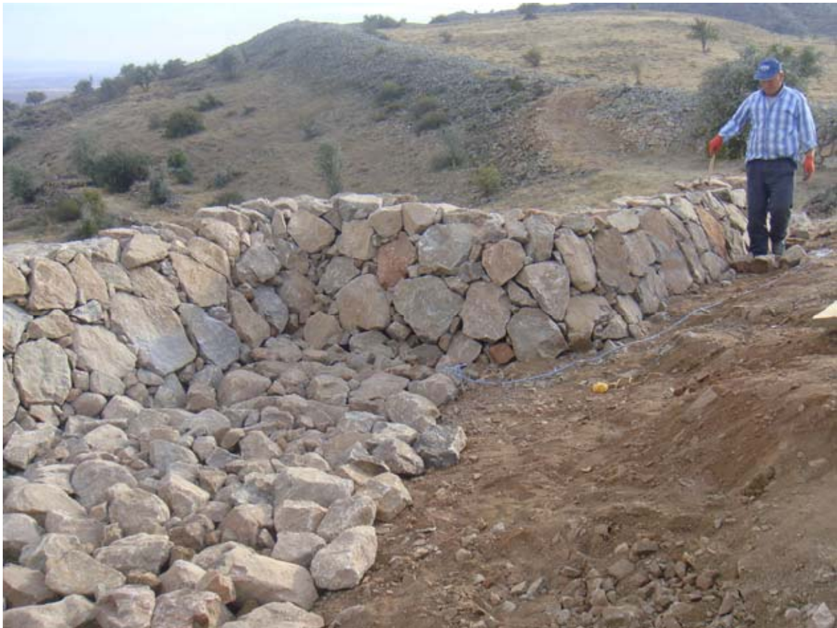
Figure 155. As a safety measure, the restored tower walls have been raised to form a parapet preventing visitors from walking too near the edge. (10dpkc3942)
