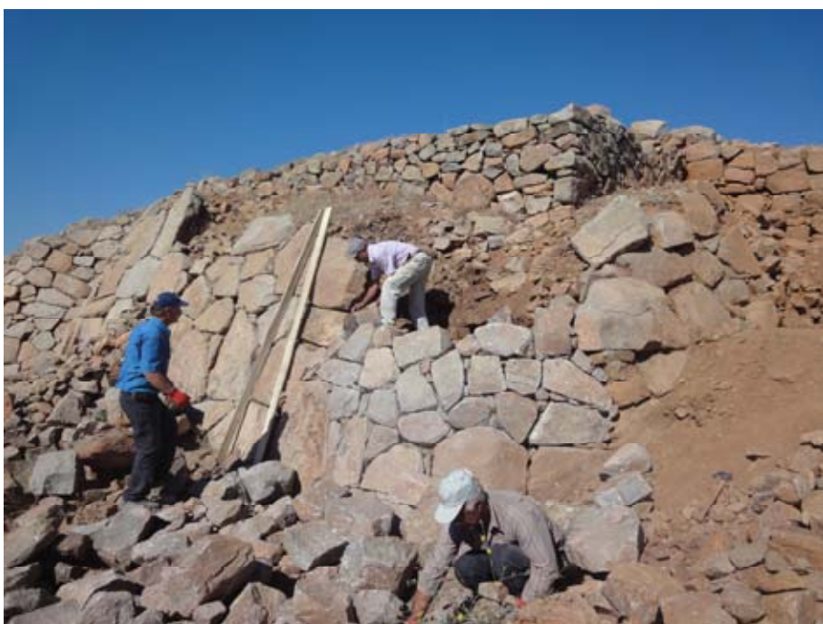
Figure 140. The east corner was restored before the remaining portion of the glacis was uncovered, thus providing structural stability and minimising the risk of further collapse. (10dpkc3302)
