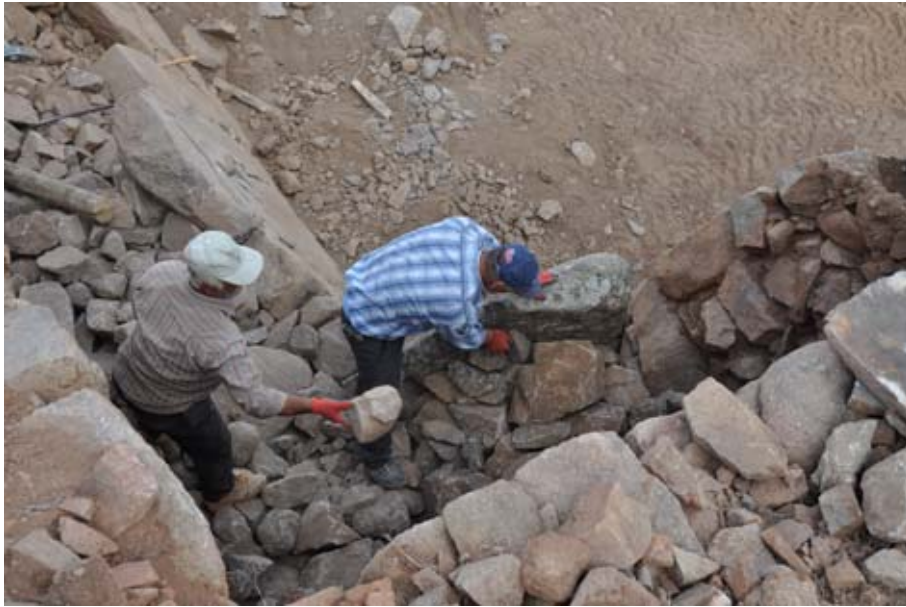
Figure 152. Small and medium stones were selected to fill up the space behind the facing stone. (10dpnd1387)
