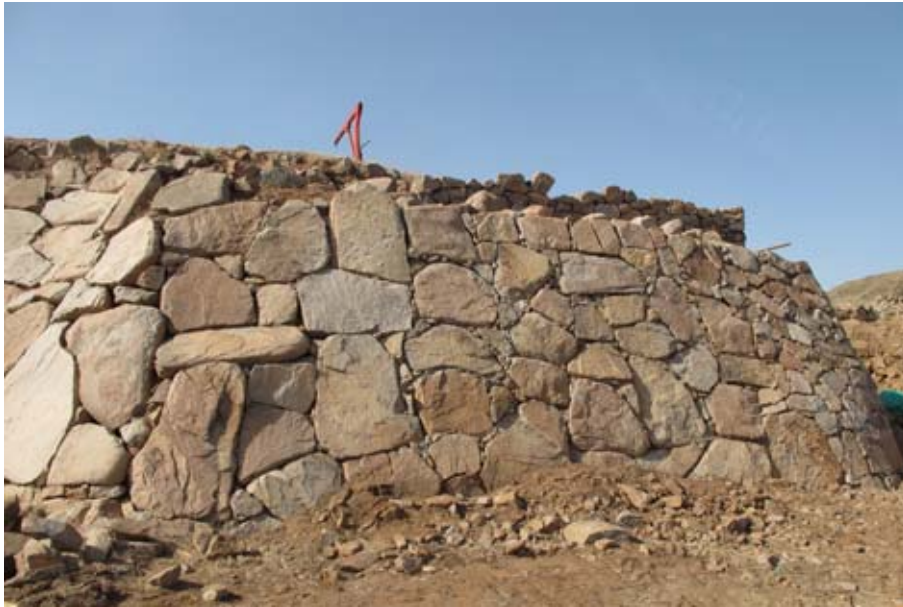
Figure 143. Once the east side of the glacis was built up to the height of the adjacent stretch of glacis, it was found necessary to relocate two slipped stones, at left, before rebuilding the top of the glacis. (10dpcg0318)
