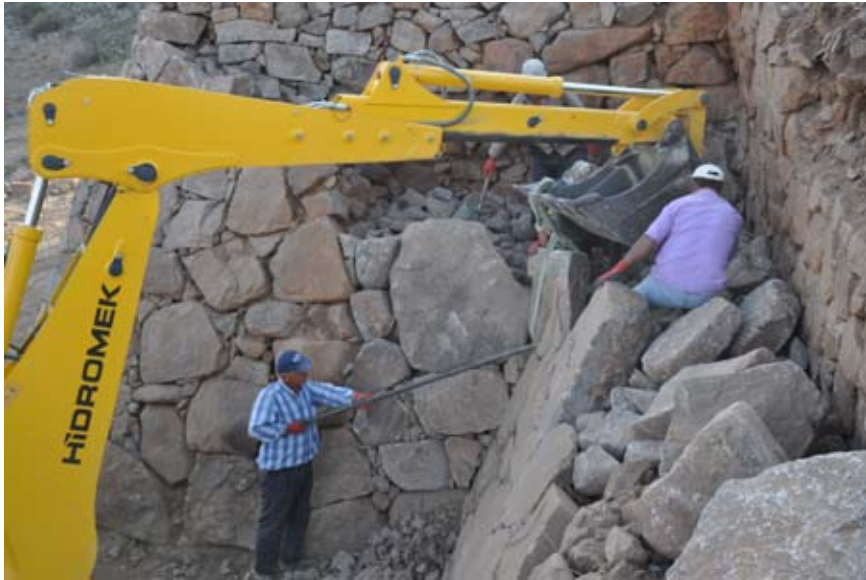
Figure 150. The machine's bucket was used to lift large and heavy stones. (10dpnd1395)
