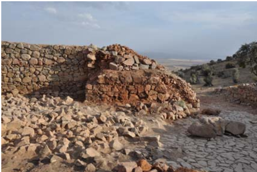
Figure 99. The wall's lack of structural stability is a result of the gap left by the horizontal timber beam after it burnt out. (10dpnd1390)
