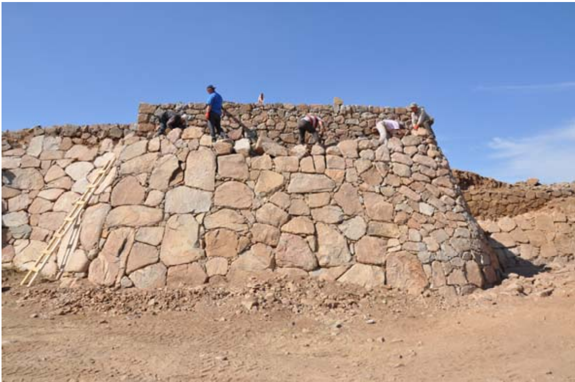
Figure 148. Once the two large stones in front of the Middle Tower were moved back to their original position it was possible to rebuild the glacis to its original height. (10dpkc1141)
